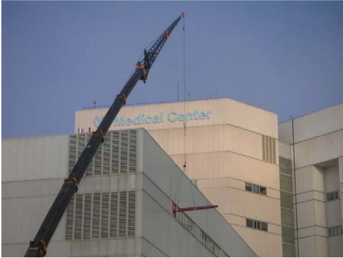
**Figure 7: Installation of (N) BRBF's at VA Seattle through upper-story window**
