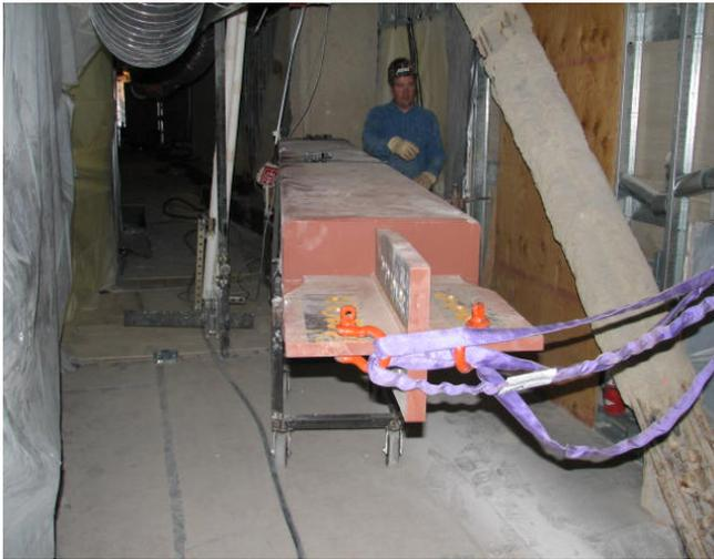
**Figure 8: Replacement of (E) TS's with (N) BRBF's at VA Seattle**
